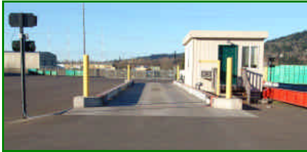
Incoming and outgoing trucks use these scales
