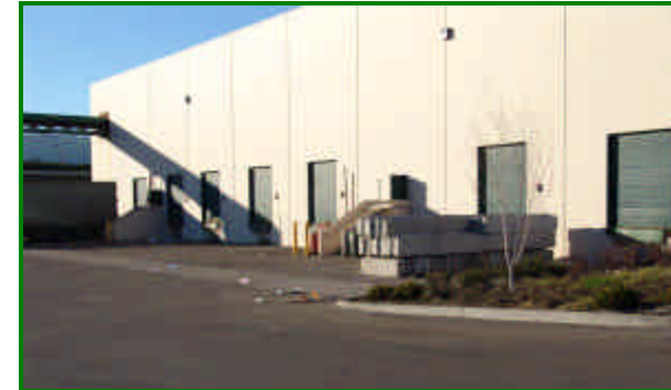
Departing trucks load recycled materials at these docks
